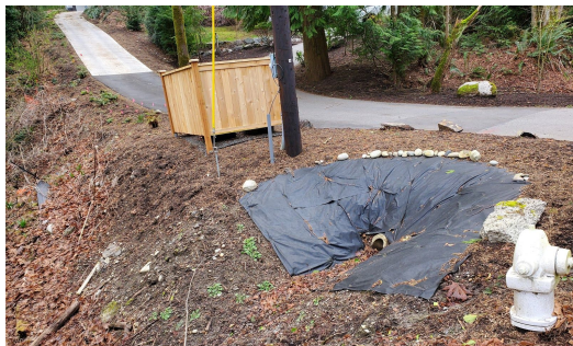
Photo 3: Black tarp around a pipe
