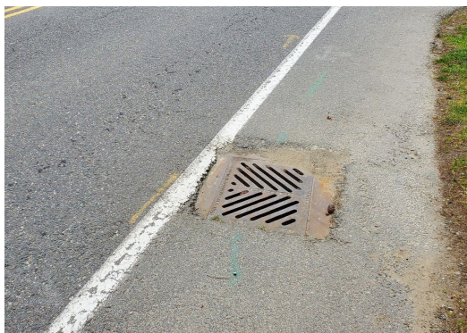
Photo 4: Storm drain on the side of the road
